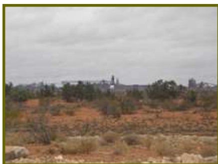
Olympic Dam main shafts 2009
